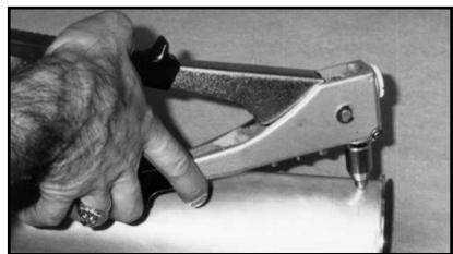
**Step 14:** Using only the factory supplied pop rivets, apply a good amount of the Seals-All Sealant around the base of each pop rivet before installing into each of the four holes. Using the pop rivet gun, permanently fasten the A1100 riser collar to the top of the drop tube.
