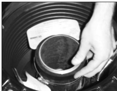
**Step 19:** Use the hose clamp to clamp the warning plate (p/n 564420, supplied), onto the riser pipe below the threads. Make sure label is facing up.
